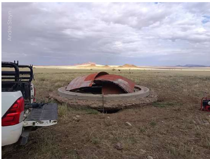
The dismantled Zebra dam.
