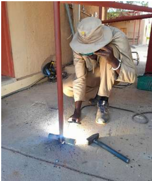
Welding the playground frame.
