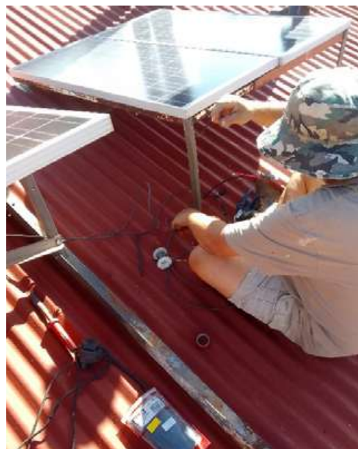
Mr Martin replacing panels at one of the Family Hideout Camps.
