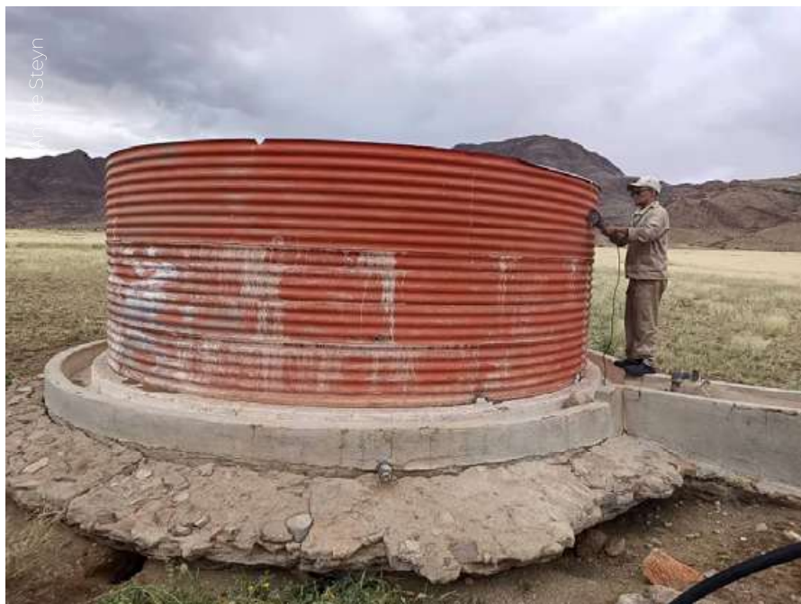
Elton busy cutting the old Zebra dam apart, using an angle grinder.
