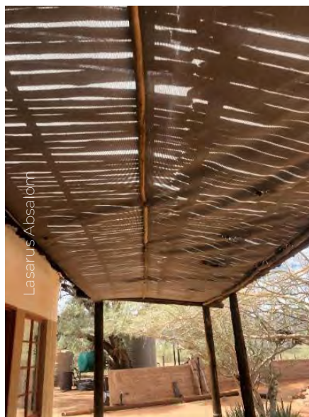
The new veranda
