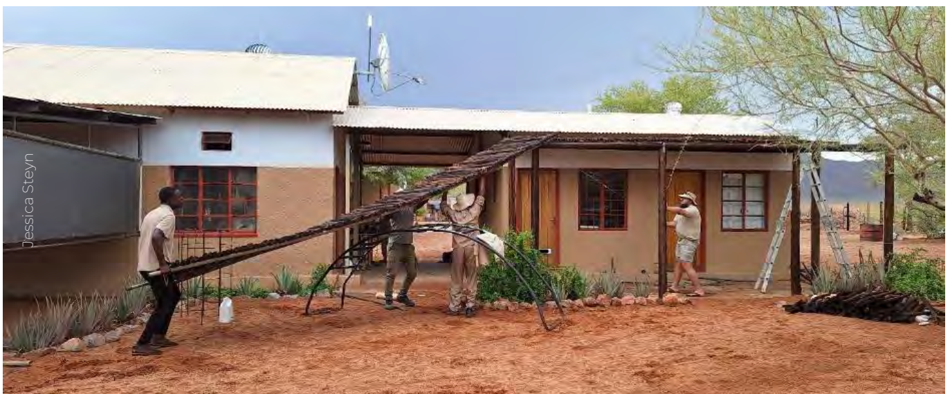
Staff installing the new veranda
