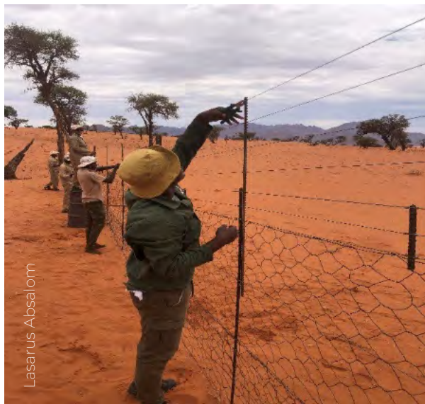
Working on the fence line
