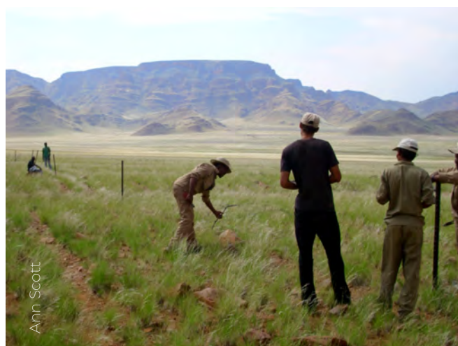
Fence removal between Vreemdelingspoort and Geluk in 2011
