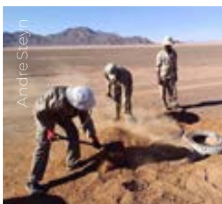
Digging in the tyres on the airstrip
