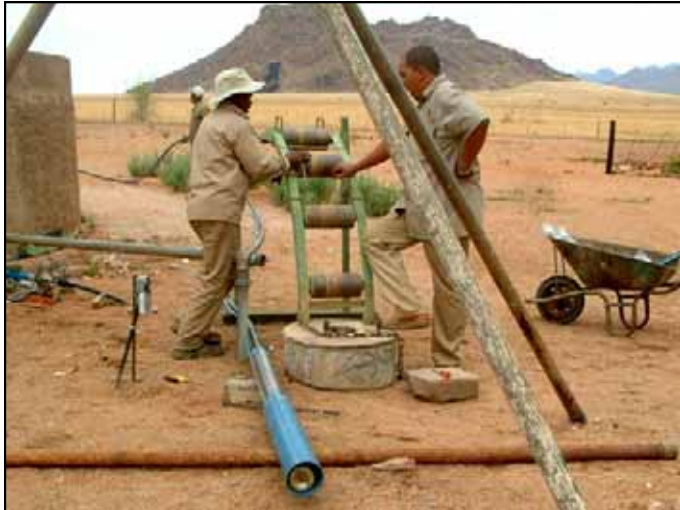
The Grunfos pump (in blue protective sheath) ready to be replaced down the 165m Keerweder borehole.
