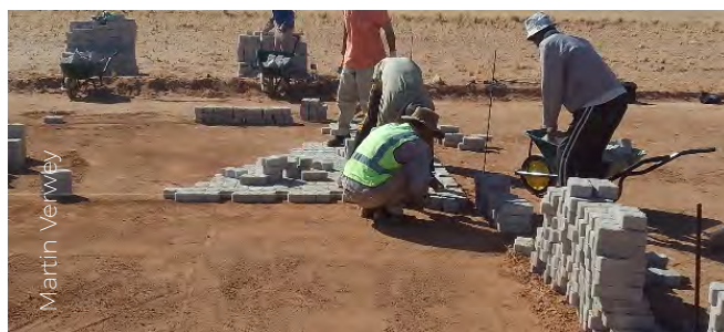
Placement of the first pavers
