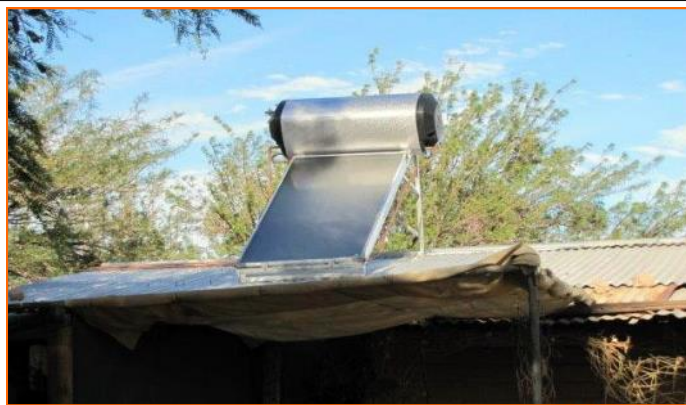
Top: The new solar geysers installed at the staff houses.
