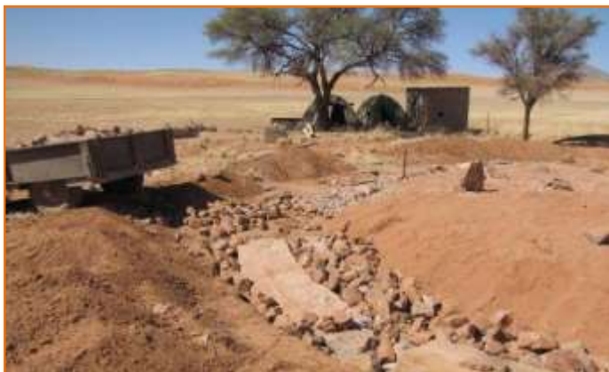
Top: The work done on Grootpomp.
