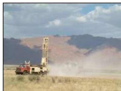
Hammerstein Drilling, hard at work on the new Keerweder borehole.
