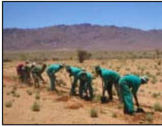
Digging of Bobbejaan-Keerweder pipeline
